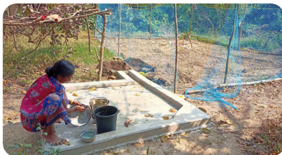
Platforms constructed to drain out greywater into Nutrigarden
