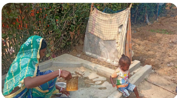
Platforms constructed to drain out greywater into Nutrigarden
